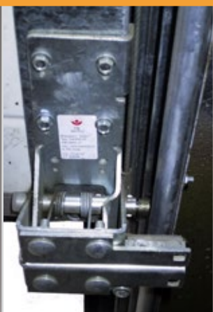
steel line break protection (MZL)
